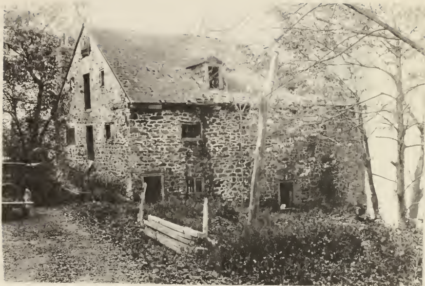
Figure 72. Latest known view of mill prior to its demolition in 1929. This photograph reveals the deteriorated condition of the building. (Mill Grove Files, Audubon, PA)
